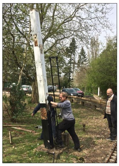
Planted in the 1960's the somersault signal post has succumbed to irreparable rot. A detailed technical examination (wobbling it!) showed it to be very unsafe. Rather than contrive ungainly temporary props a decision was taken to remove it without delay. Removal as can be seen in the picture above required little more than a shove and down it came. Timber for a replacement, supplied with the correct 8" to 7" taper has been located. Les B
